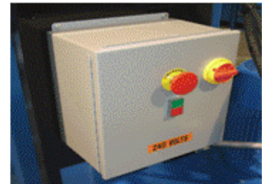
Electrical control box NEMA- 12 Key lockout, Emergency stop push button. Dust, oil and rain prevent with occasional wash down.
